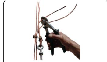
After complete hogging and fine adjustment (red and yellow) cut the unnecessary hanger robe.
