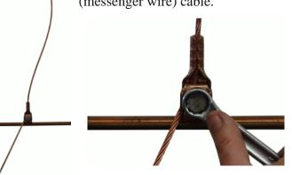
**5.** Definite adjustment of the contact wire height. After loosening the crew, set the contact wire to the specified height by pulling at the catenary wire end.
