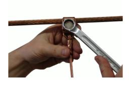
**3.** Install the compressed cable dropper clamp at the catenary (messenger wire) cable. Tighten the bolt with a torque wrench of 25 Nm.
