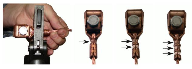
**2.** Install the compressed cable dropper clamp provisionally at the catenary (messenger wire) cable.
