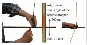
**6.** Install the cable dropper clamp at the contact wire. Tighten the bolt with a torque wrench of 25 Nm.
