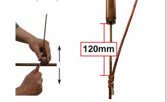
**6.** Compress the cable dropper clamp.
