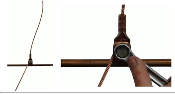
**5.** Install the cable dropper clamp definitively at the contact wire. Tighten the bolt with a torque wrench of 25 Nm.
