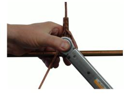
7. Cut the overlength of dropper wire.
